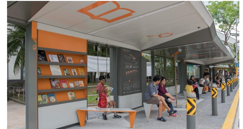
Bus stop in Singapore, Infocomm Media Development Authority.
