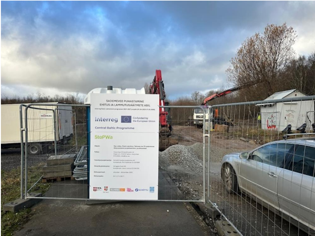
Figure A1. StoPWa project billboard during the construction phase at the Estonian pilot site.
